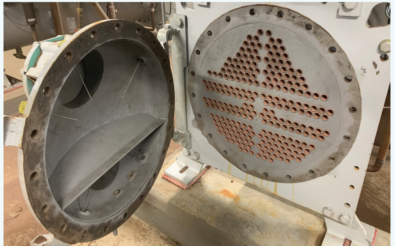
Surface after abrasive blasting - Surface preparation
