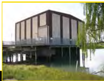
Murray Bridge Pump House
